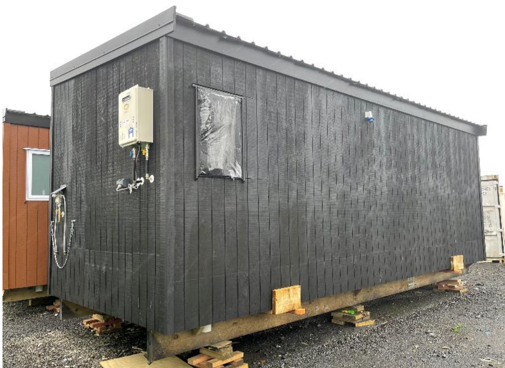
Photo 2: External elevations general view.
