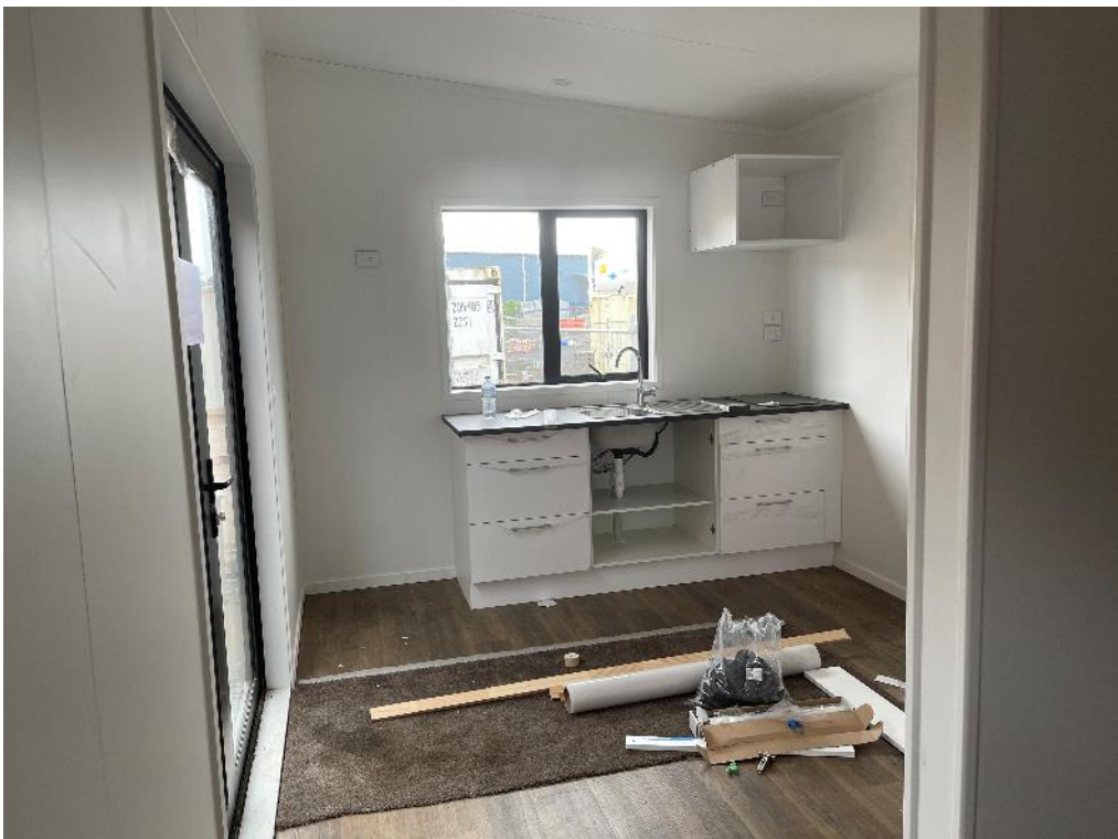
Photo 3: Lounge / Kitchen Area.
