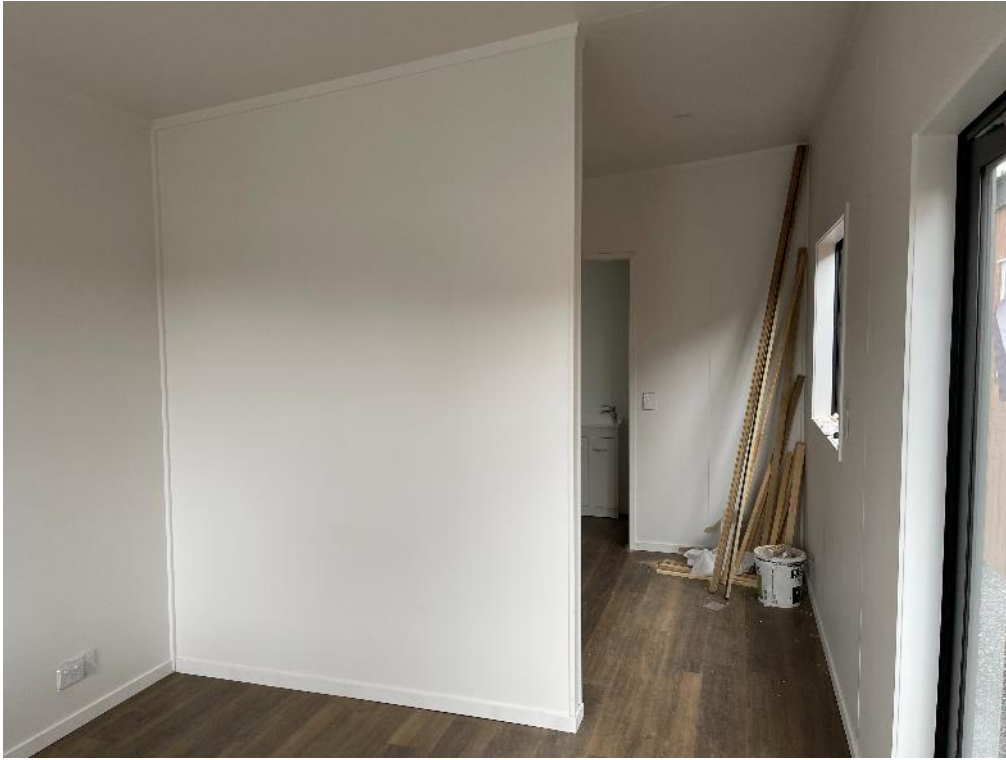
Photo 5: Lounge / Kitchen Area.
