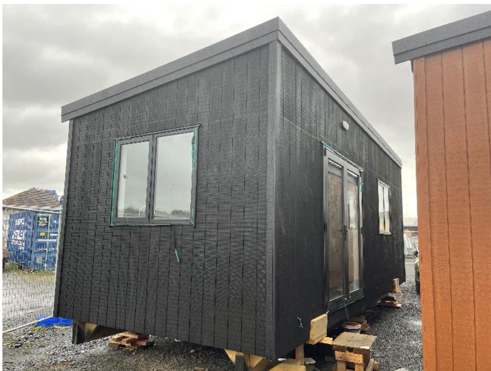
Photo 1: External elevations general view.
