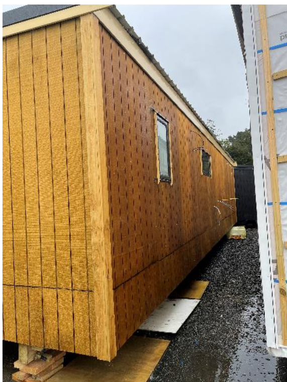
Photo 3: External elevation general view.
