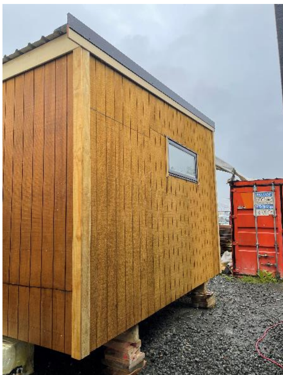
Photo 4: External elevation general view.
