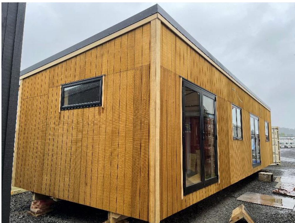
Photo 1: External elevations general view.
