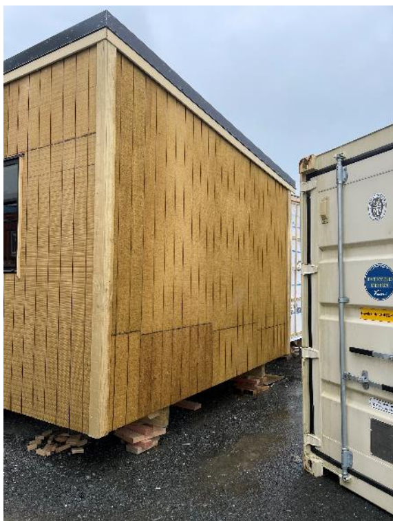
Photo 2: External elevation general view.
