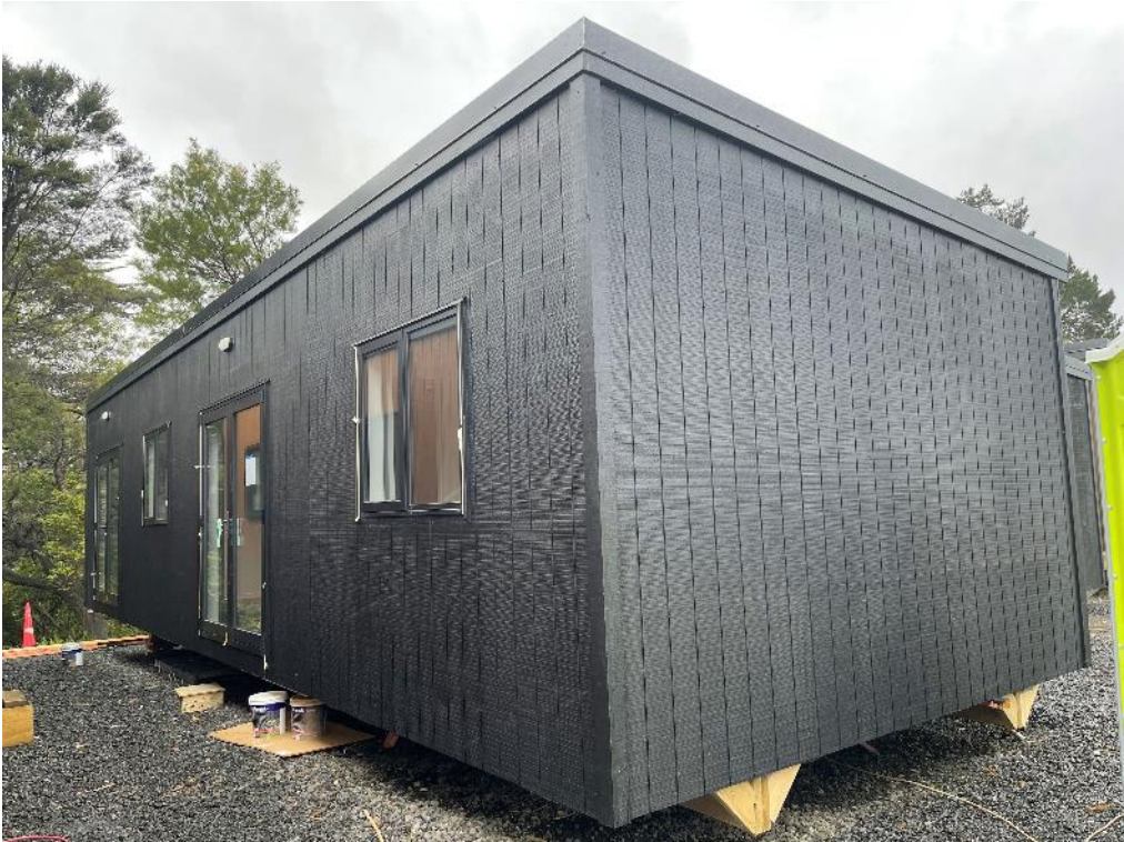
Photo 1: External elevations general view.
