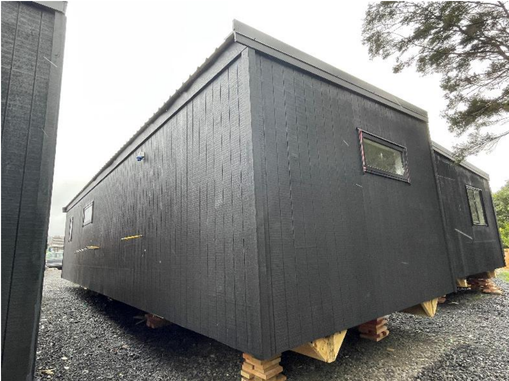
Photo 2: External elevations general view.
