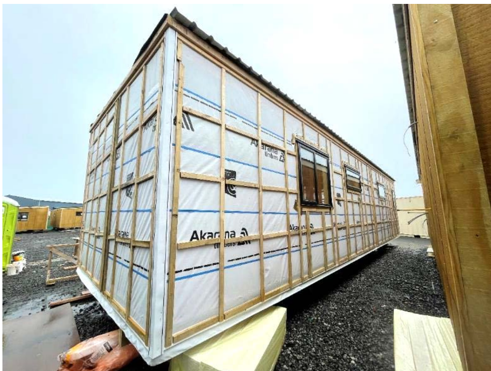
Photo 3: External elevations general view.
