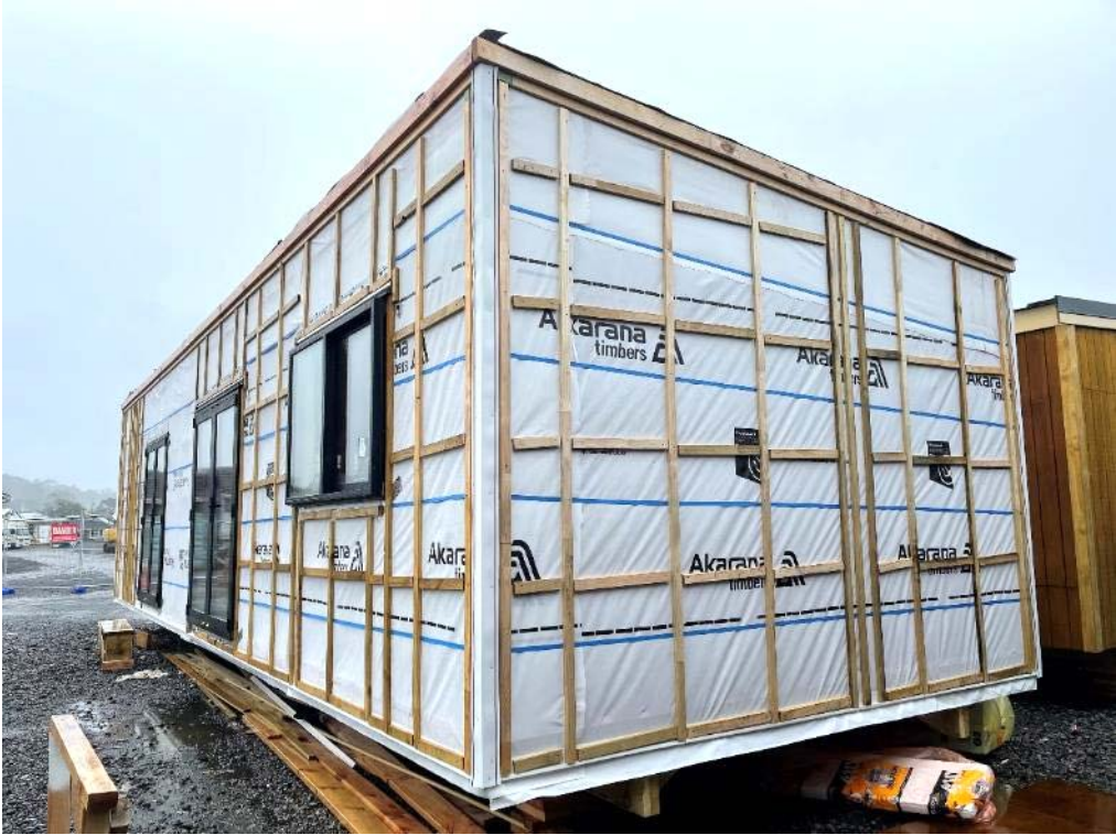
Photo 2: External elevations general view.
