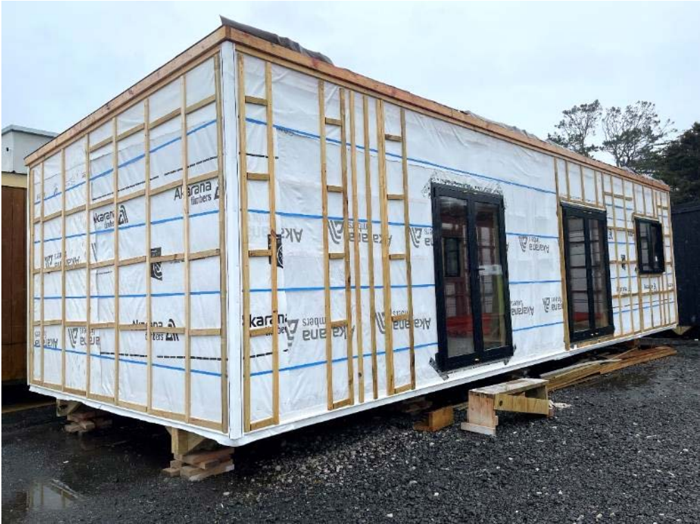
Photo 1: External elevations general view.
