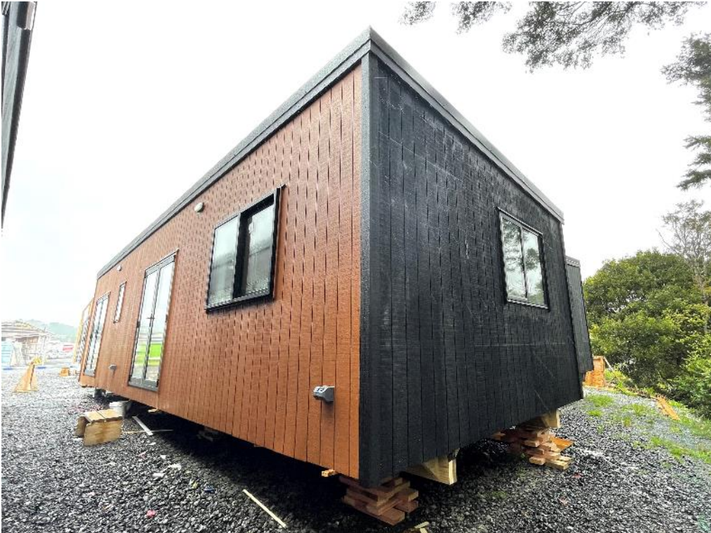
Photo 2: External elevations general view.
