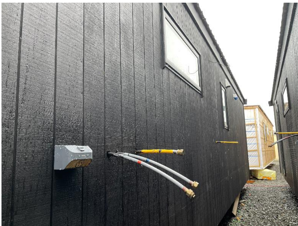
Photo 4: External elevation general view.
