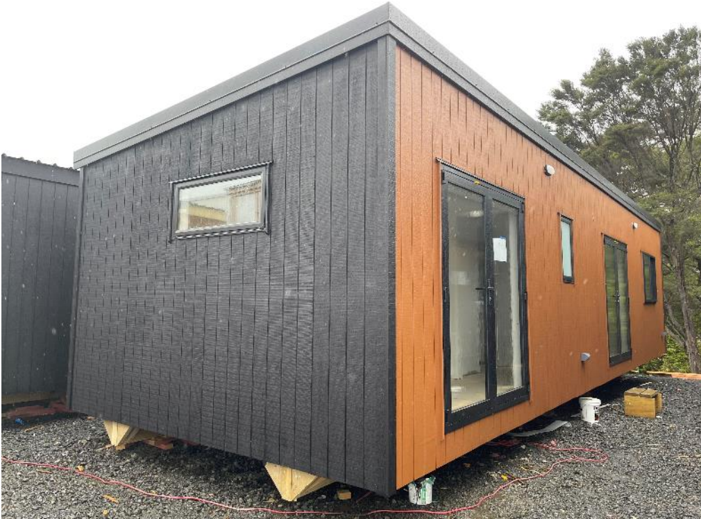
Photo 1: External elevations general view.
