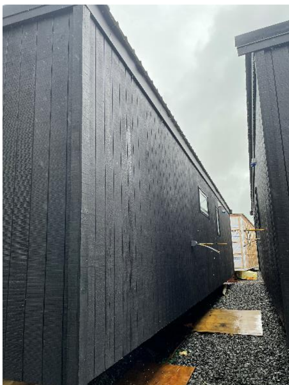
Photo 3: External elevation general view.
