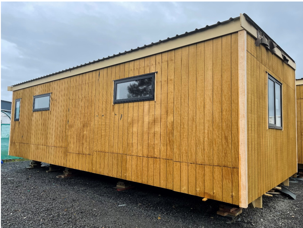
Photo 4: External elevations general view.
