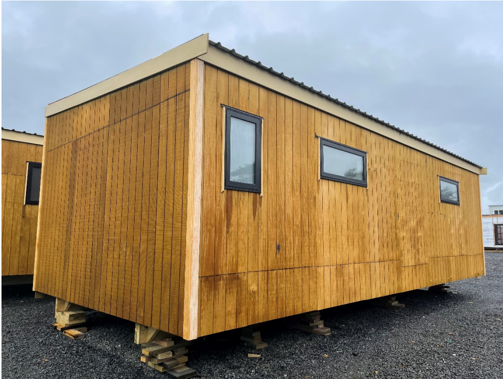
Photo 3: External elevations general view.
