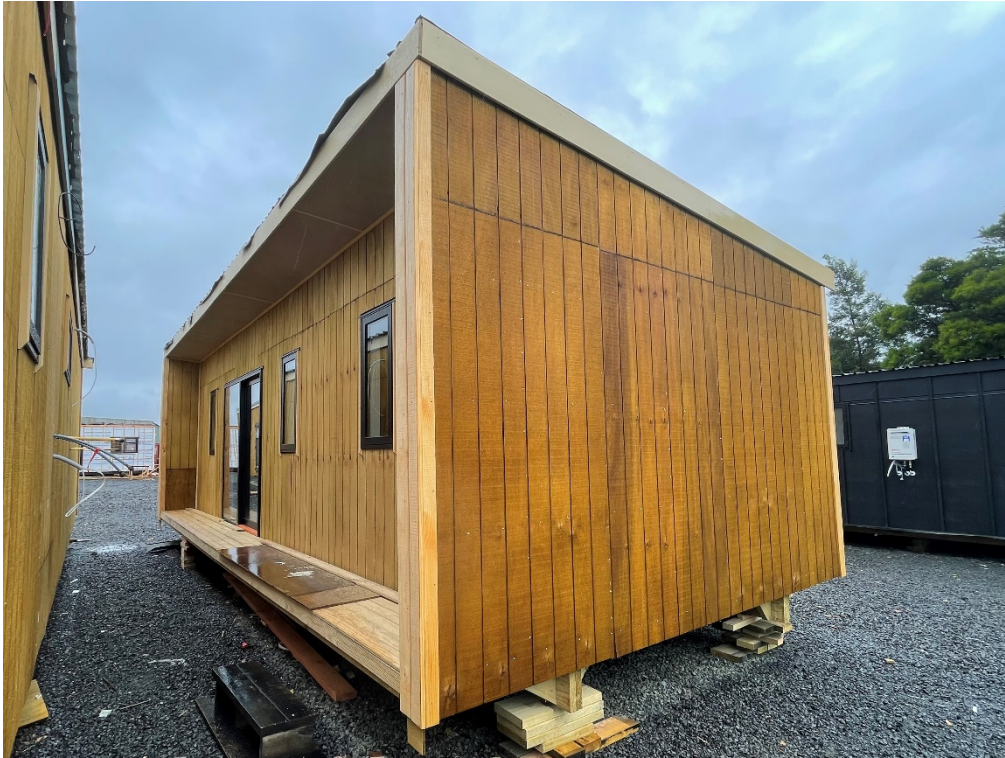
Photo 1: External elevations general view.
