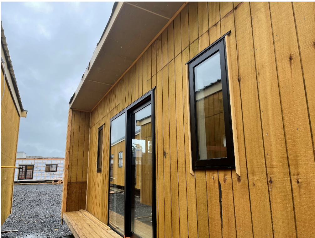
Photo 2: External elevation general view.
