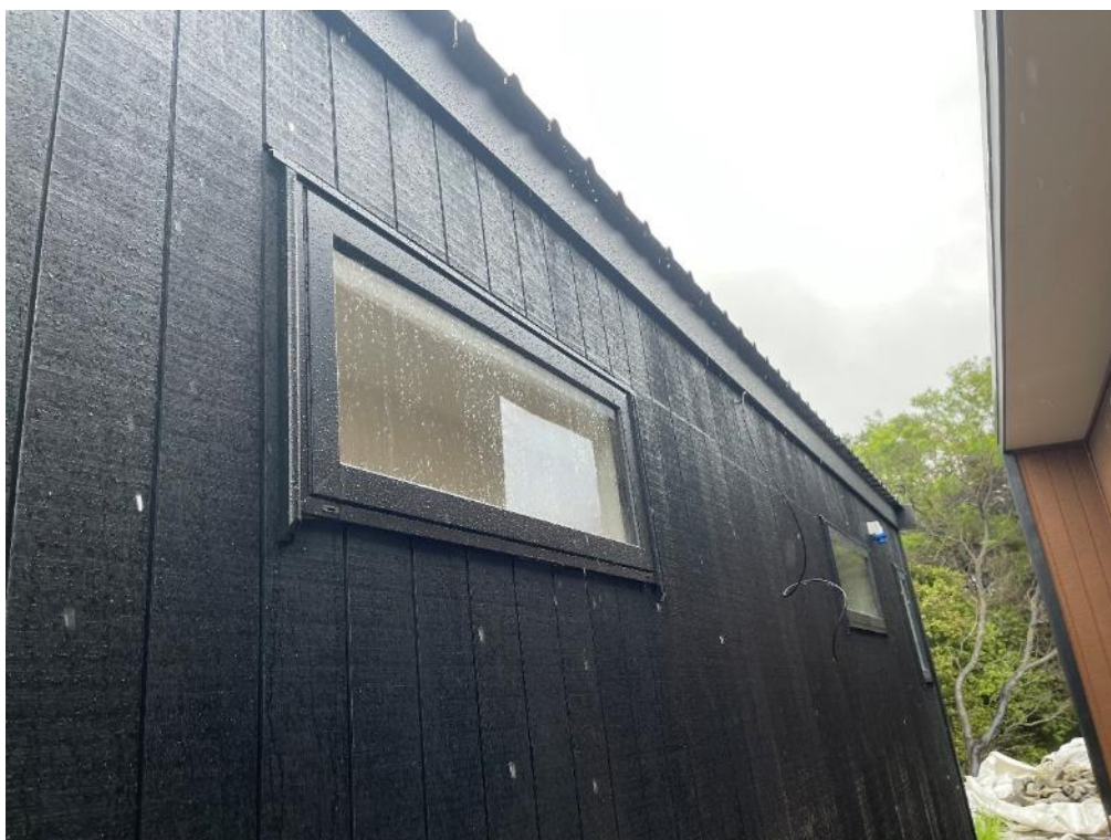
Photo 4: External elevation general view.
