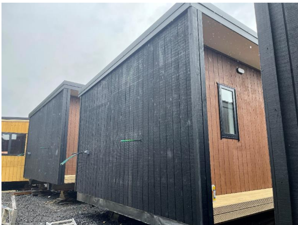
Photo 2: External elevations general view.
