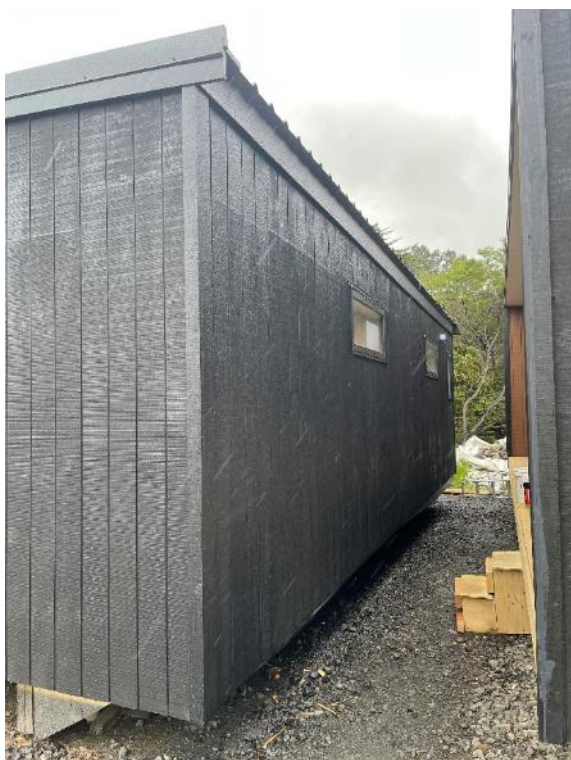
Photo 3: External elevations general view.
