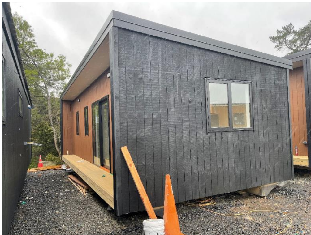
Photo 1: External elevations general view.
