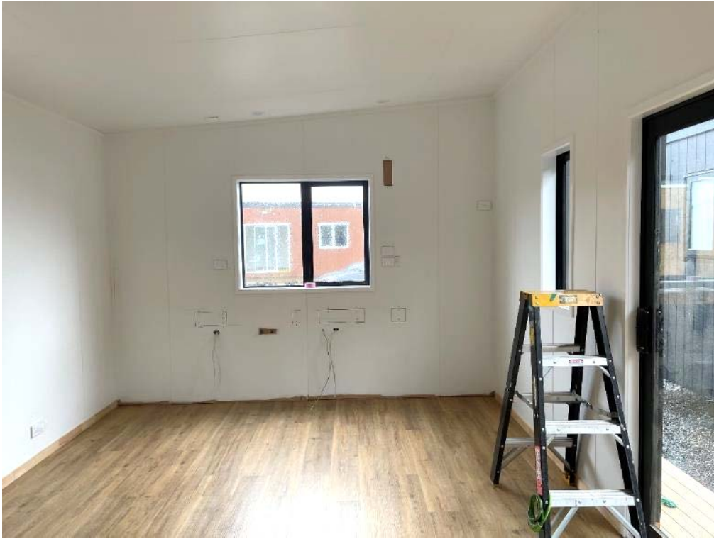
Photo 5: Kitchen / Lounge Area.
