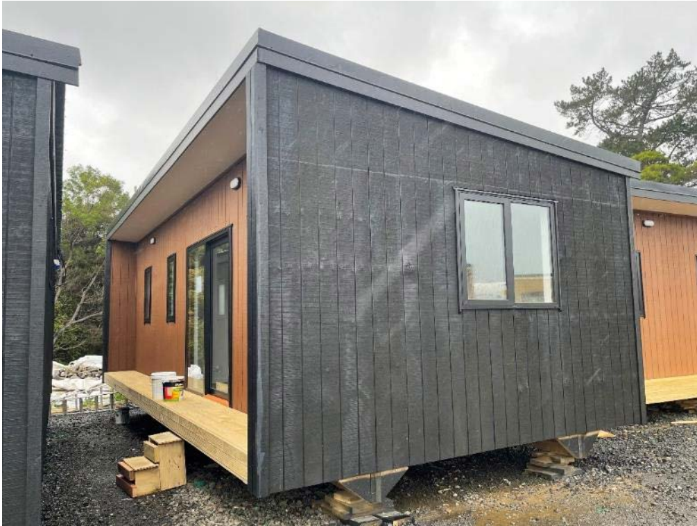
Photo 1: External elevations general view.
