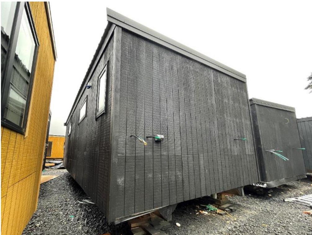
Photo 2: External elevations general view.
