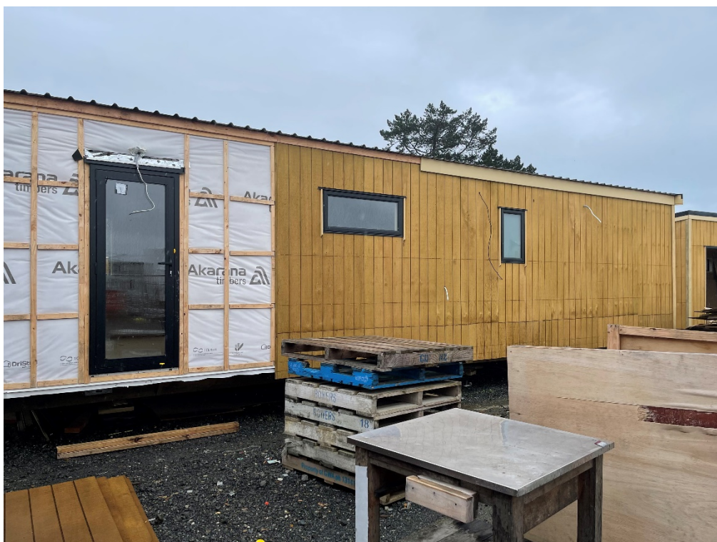
Photo 4: External elevation general view.
