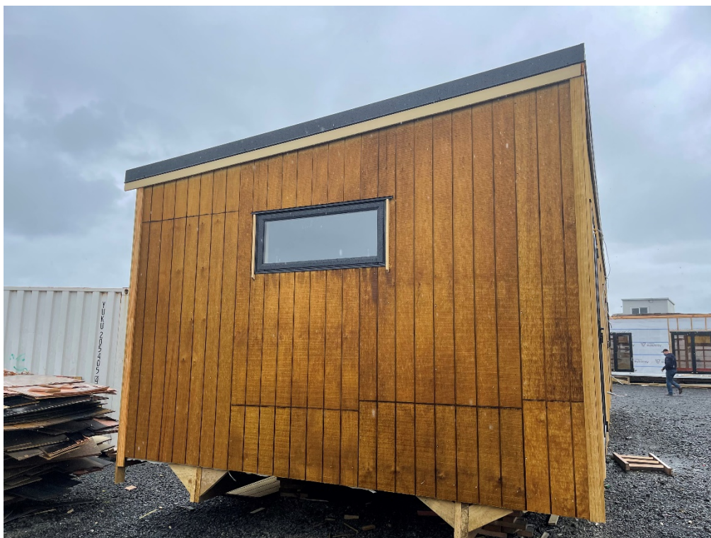
Photo 3: External elevation general view.
