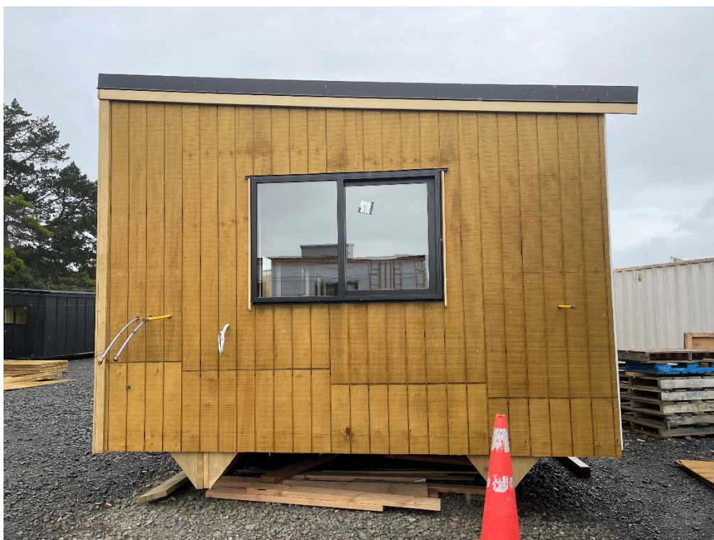
Photo 2: External elevation general view
