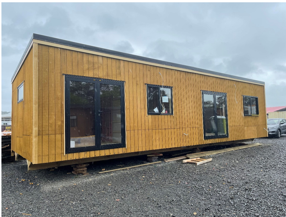
Photo 1: External elevations general view.
