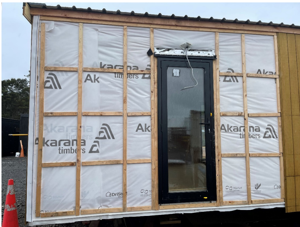
Photo 5: External part elevation general view.
