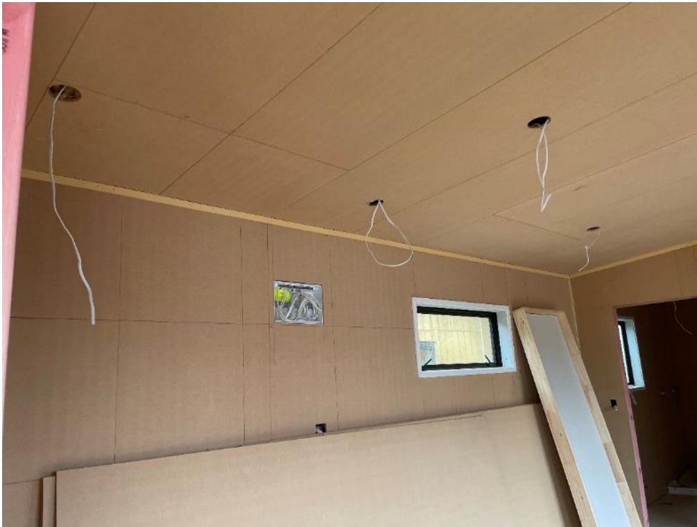
Photo 11: Lounge / Kitchen Area.
