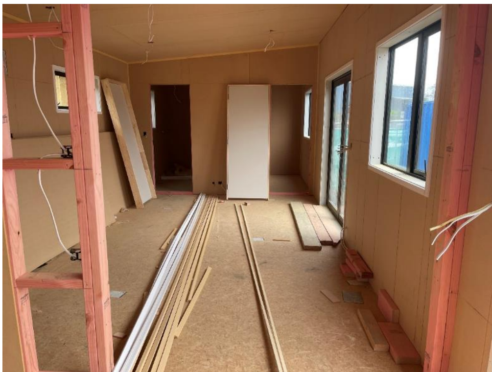
Photo 9: Lounge / Kitchen Area.
