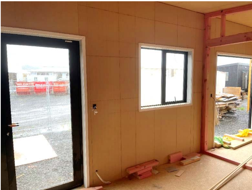
Photo 12: Lounge / Kitchen Area.
