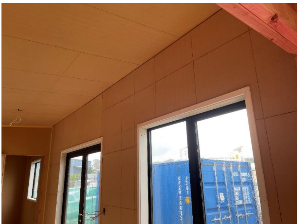
Photo 10: Lounge / Kitchen Area.
