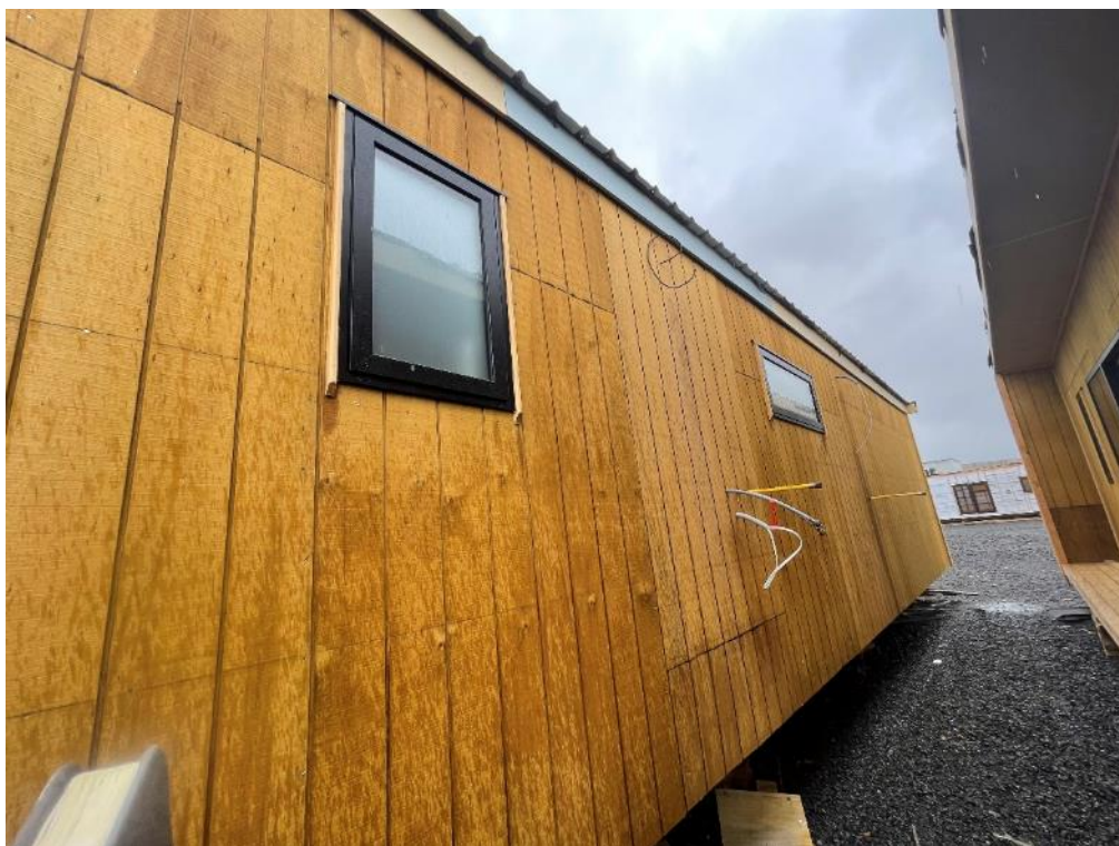
Photo 3: External elevation general view.
