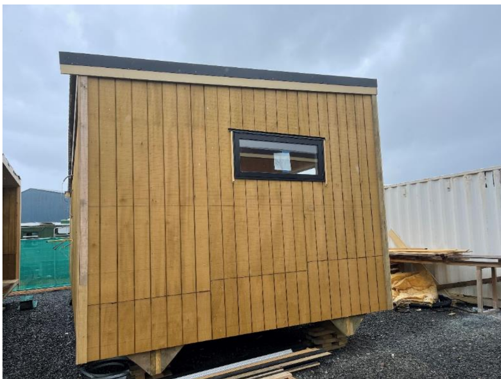
Photo 2: External elevation general view.
