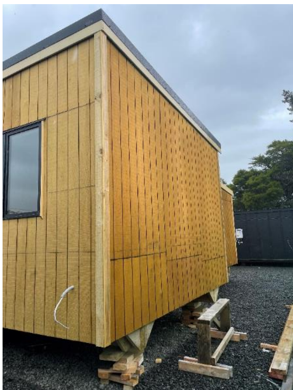
Photo 4: External elevation general view.
