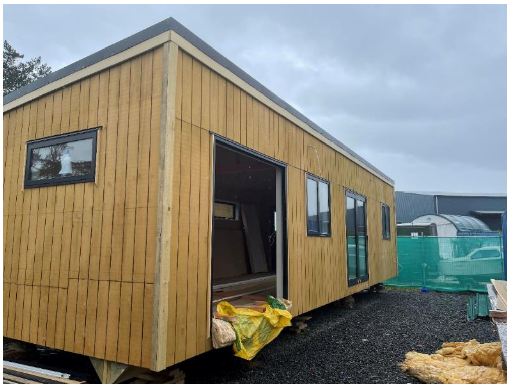
Photo 1: External elevation general view.
