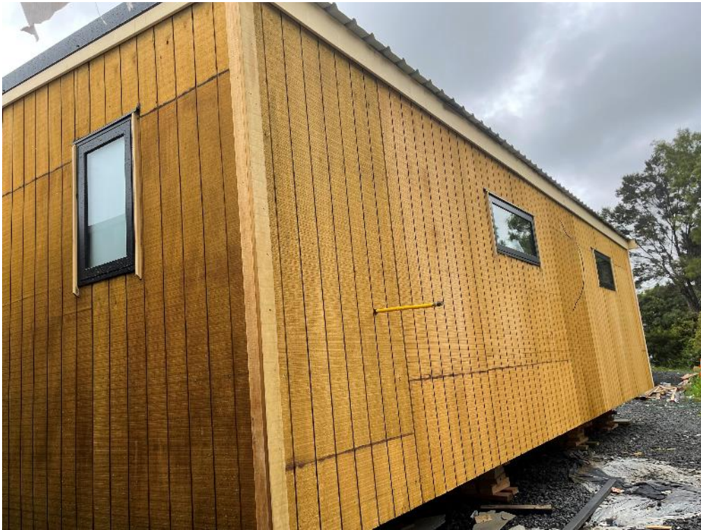
Photo 3: External elevation general view.
