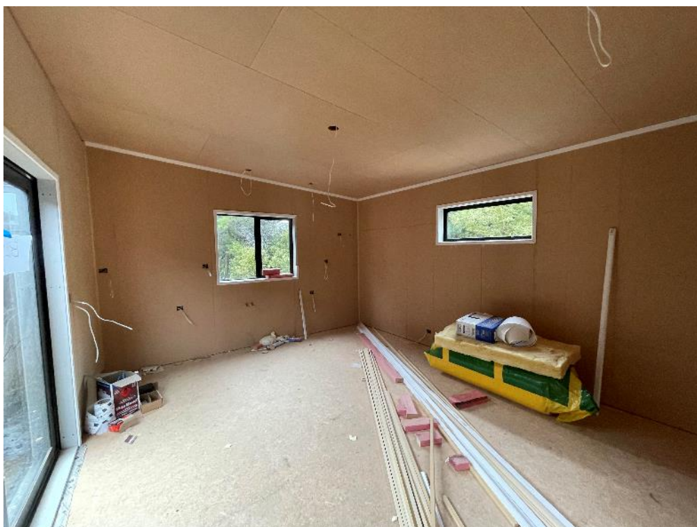
Photo 12: Lounge / Kitchen Area.
