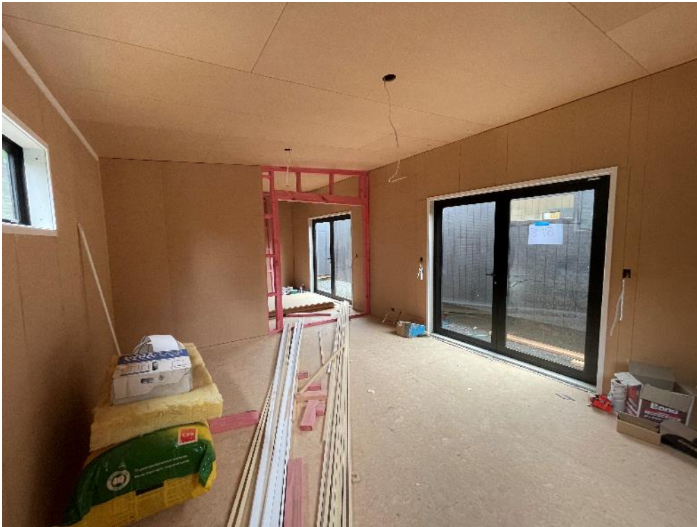
Photo 13: Lounge / Kitchen Area.
