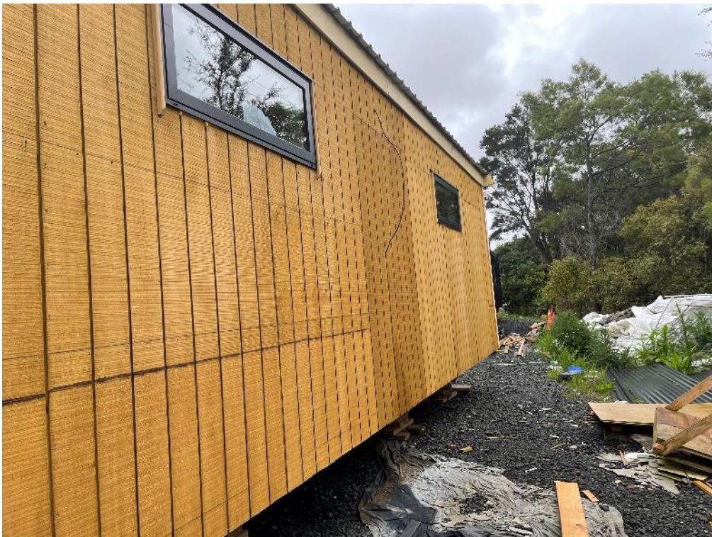
Photo 4: External elevation general view.
