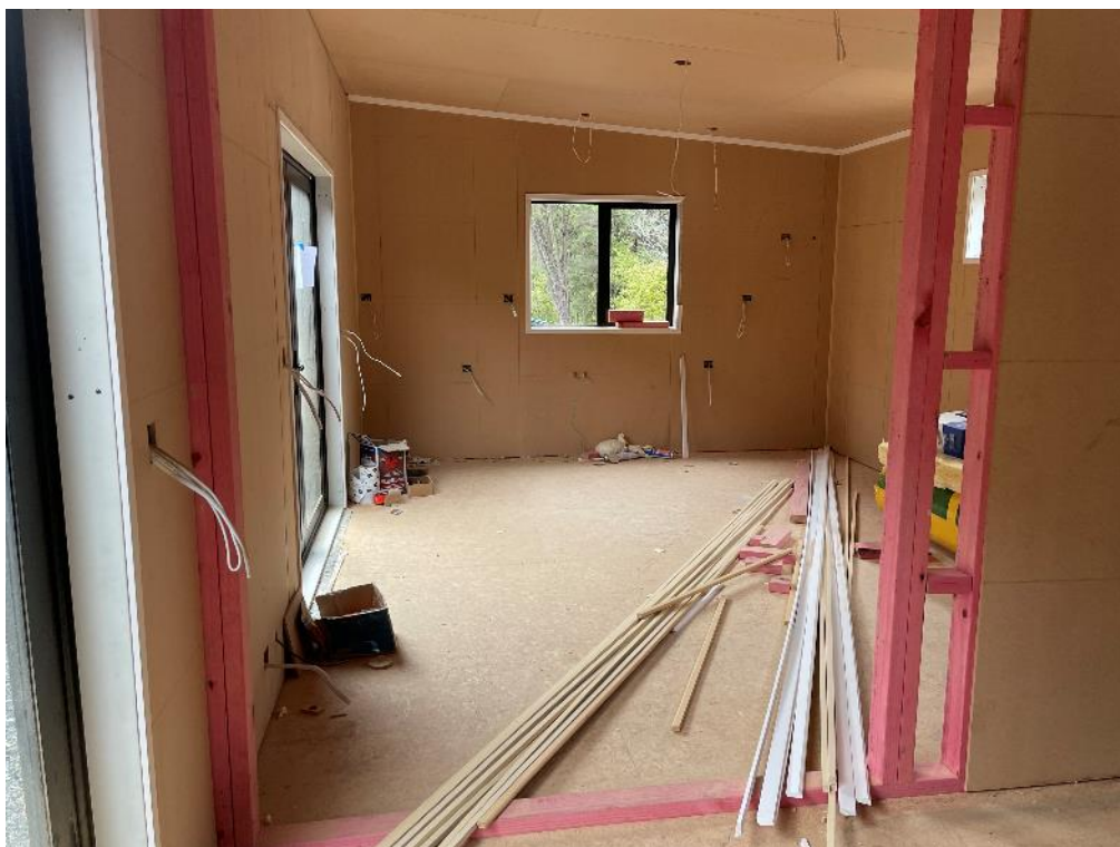
Photo 11: Lounge / Kitchen Area.
