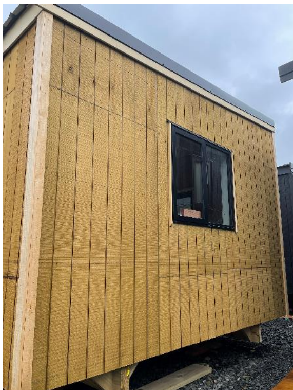
Photo 2: External elevation general view.
