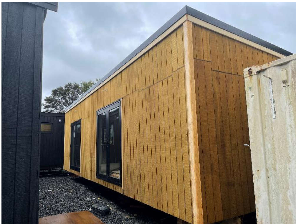
Photo 1: External elevation general view.
